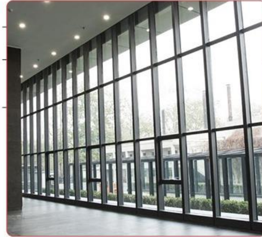
Glass Curtain Wall
